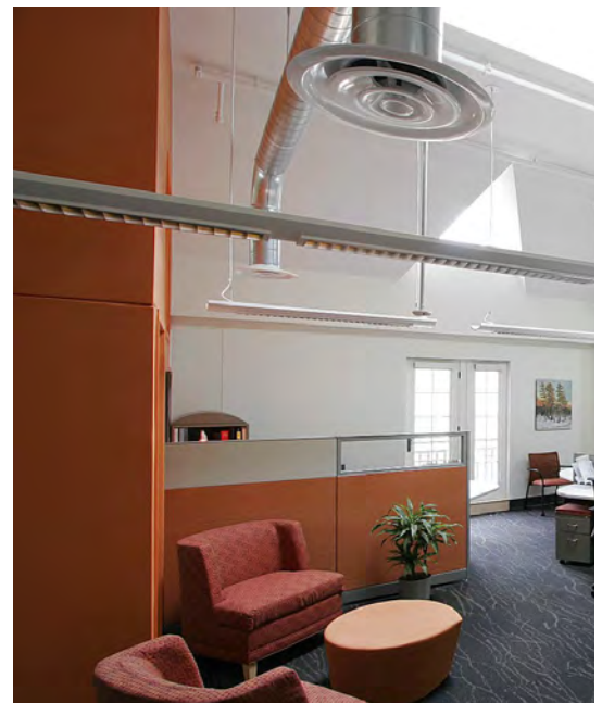
Exposed spiral ducts can be installed in existing spaces or new construction. Photo © Maclay Architects
